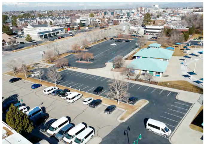
SCERA Pool: Existing Parking & Facilities
