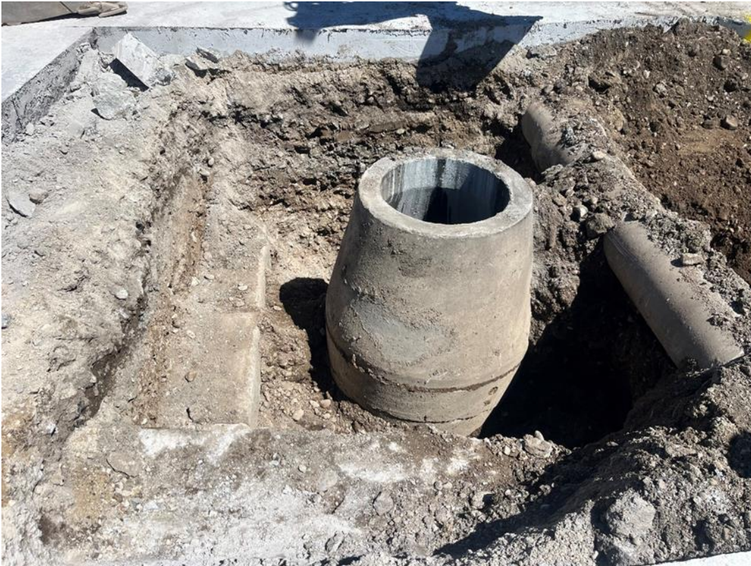
900 South Sewer Replacement Project
