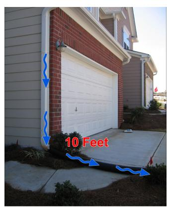
protects the building foundation from water damage. So if roof water is intended to discharge near the base of the building (as many downspouts do) ensure that slope requirement is met.
