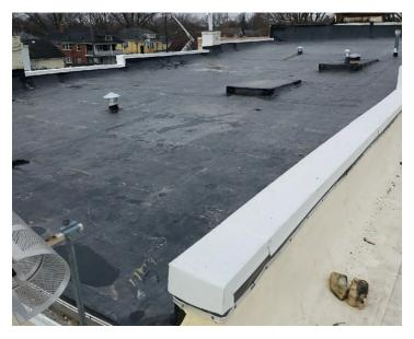
Synthetic roofing is used for waterproofing purposes and is composed of a variety of polymers. They come as flexible sheets or can be applied as a liquid directly to the roof. This style of roofing is most often used for large retail buildings and commercial structures. Pollutants found in roof run-off from synthetic roofs include inorganic substances, organic contaminants, and nutrients. Zn, As, Ba and harmful inorganic compounds used as plasticizers can also be found.
