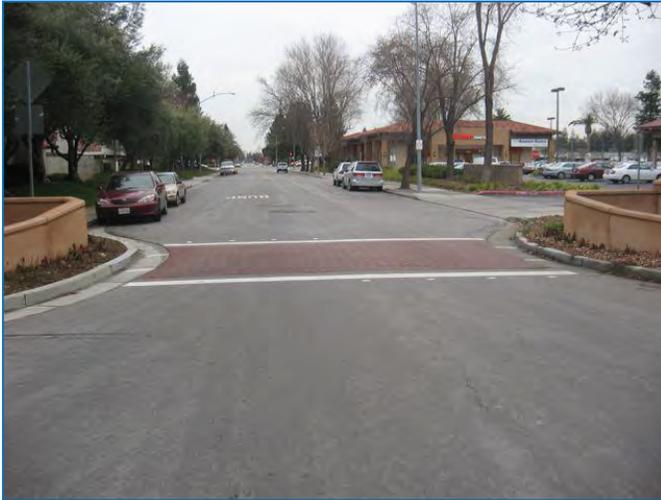
**CHOKERS** are curb extensions at mid-block that narrow the roadway by widening the sidewalk, planting strip, or centerline. A typical two-lane choker is 20 feet from curb to curb. One-lane chokers narrow the roadway to just one travel lane. This is similar to a one-lane bridge condition. The constricted length in the direction of travel varies but should be kept short enough not to block the driveways or accesses.
