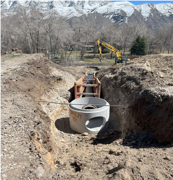
400 South Storm Water
