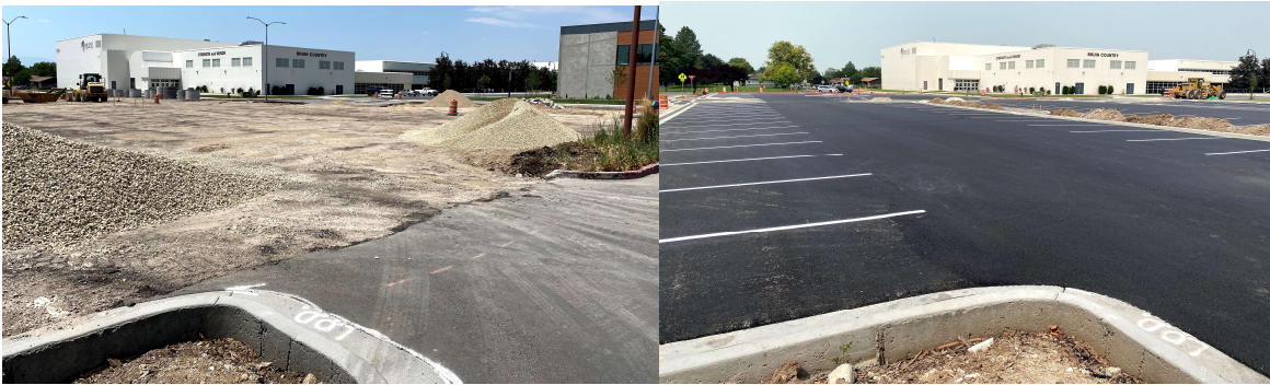
Debris Flow Mitigation Project
