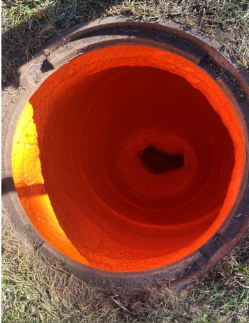
Sewer Rehabilitation Project
