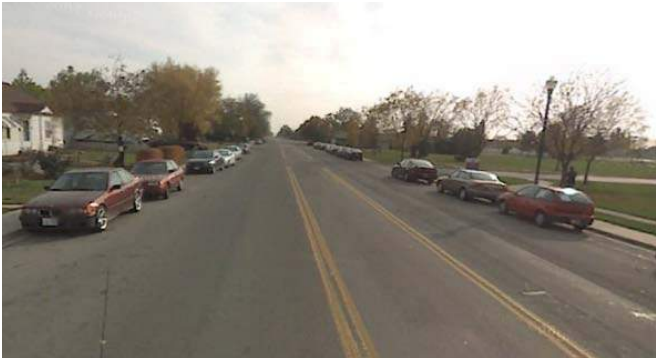
400 West near 310 North
