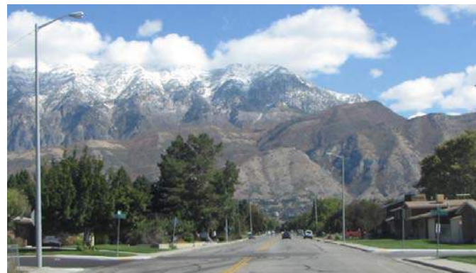
Wide roadway with no supplemental striping on E 400 North
