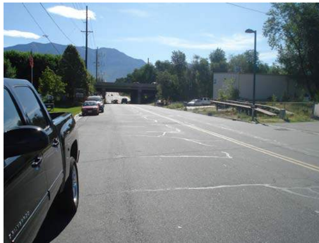
A facility barrier is exemplified by lack of pedestrian sidewalks on 400 South (west of I-15).
