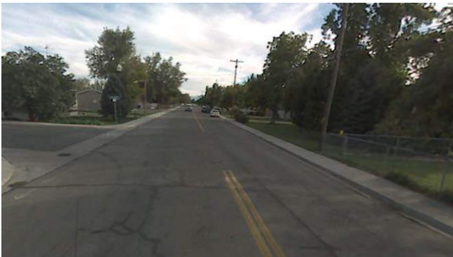
400 West near 580 North
