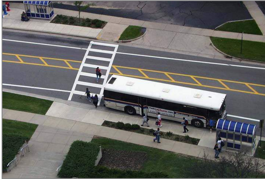
Complete Streets are designed for all users (image: Complete Streets Coalition – www.completestreets.org )
