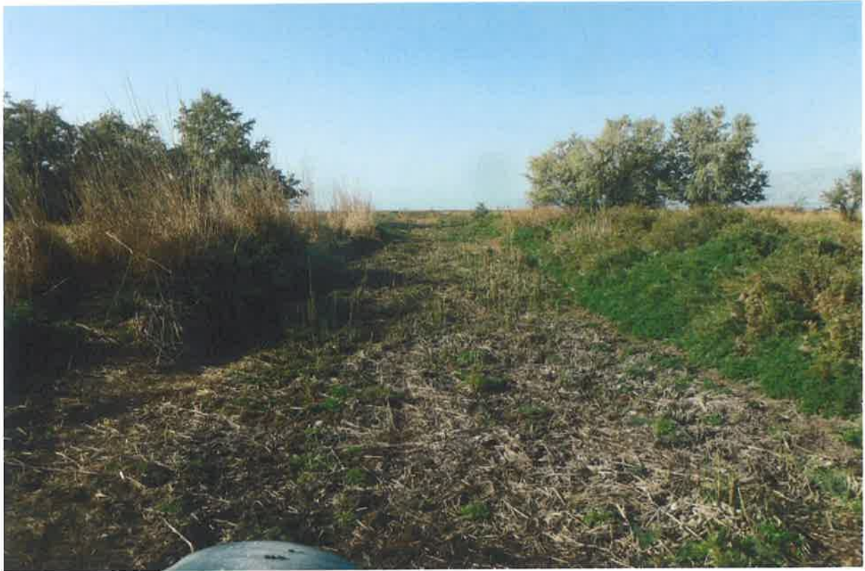
Photo 2. Taylor Ditch looking West into Utah Lake. (10/5/20).
