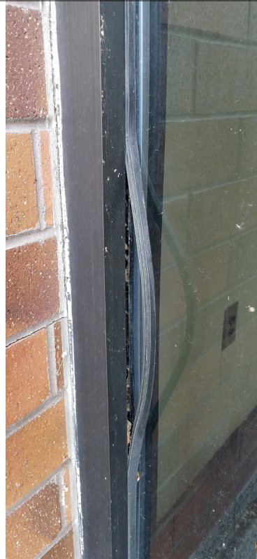
Several of the storefront systems are missing their insulating glass seals and have been replaced with caulk which may be causing unnecessary heat gain or loss.
