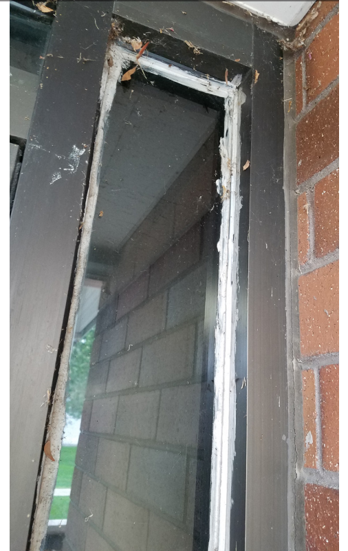
Several of the storefront systems are missing their insulating glass seals and have been replaced with caulk which may be causing unnecessary heat gain or loss.
